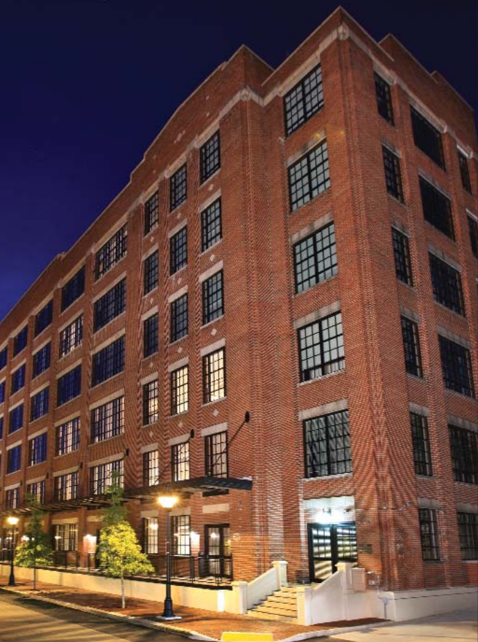
The River Lofts III, located along Richmond's Tobacco Row, houses 131 luxury apartments.
